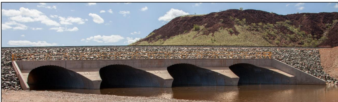
Corrugated-plate arches - Rio Tinto – RCE 333 Expansion Project, WA.
