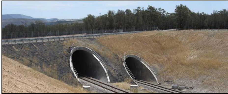
Corrugated-Plate Structures, Wambo Rail Spur, NSW
